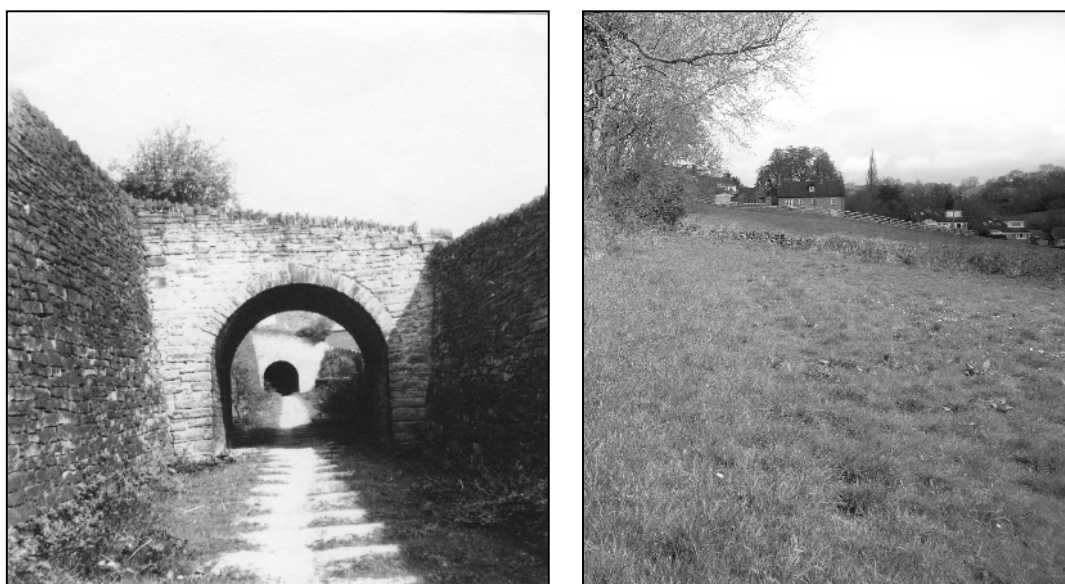
Fig.3. Comparative views of the old and new alignments looking north from just south of Fritchley village (OS Grid Ref. SK358529). The image on the left 8 was taken in 1946 and shows an occupation bridge and the tunnel in the distance on the new alignment. The right image was taken in 2014 from about 50m to the east and shows the formation of the earlier alignment.
